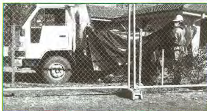
Demolition workers wearing protective clothing and masks due to the asbestos risk at Gordon. No such protective gear provided for tenants!
